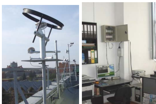
Figure 6. Station for measuring the meteorological parameters at WUT
